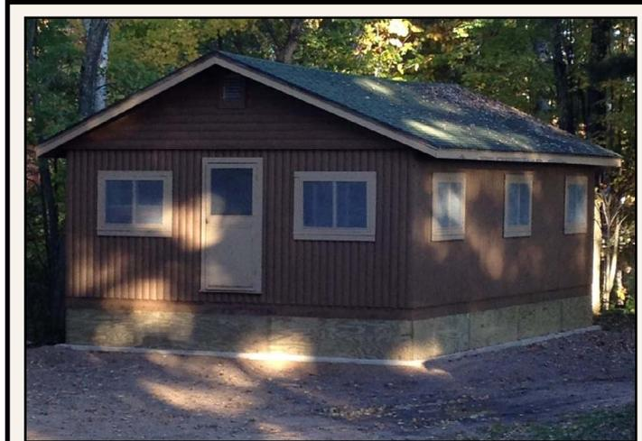
Cabin J7 gets a face lift.. with "lift" being the key word! In addition to the new coat of paint, you'll notice the new foundation. Workers came in, slid two steel beams under the cabin and lifted the whole cabin off its old base. A new foundation was poured and J7 is now resting on its new base. This is the same process that was done to J2 & J3 several years ago. Tom will put some new steps in before the campers arrive!
